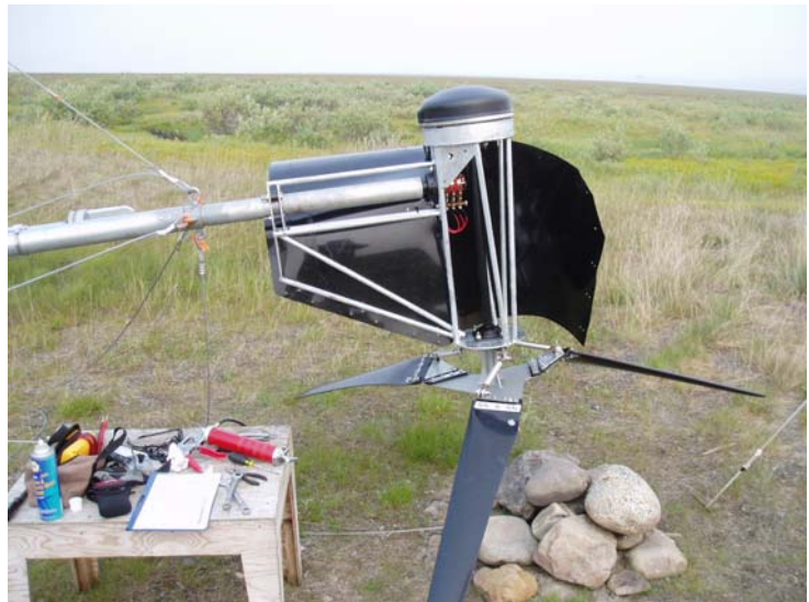
Proven turbine lowered for maintenance.
