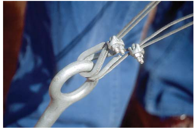
Guy cable detail: thimbles
