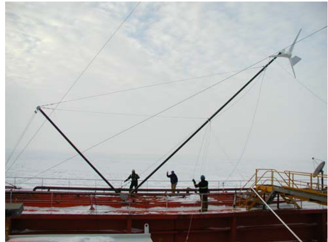
AWP installation at Beaufort.
